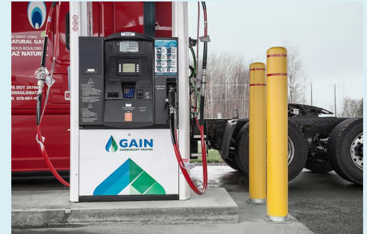
Quick fill dispenser: 5 to 10 minutes per truck
