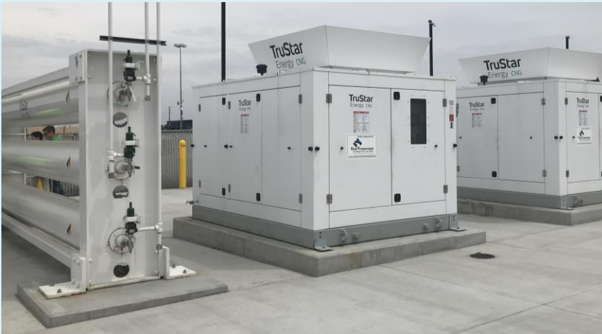
Compression equipment (station)
